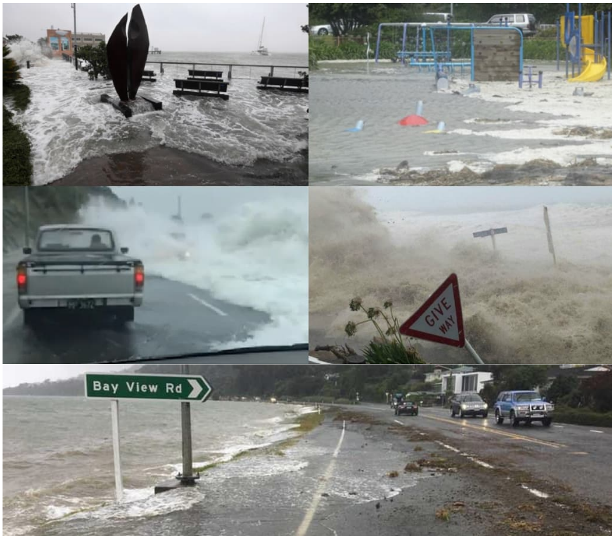
Figure 6.1: Wave runup and overtopping observed during Ex TC Fehi. (Top left) Wakefield Quay, (top right) Tahunanui Beach, (middle left) Rocks Road, (middle right) Seafield Terrace, The Glen, (bottom) Bay View Road, Atawhai.
