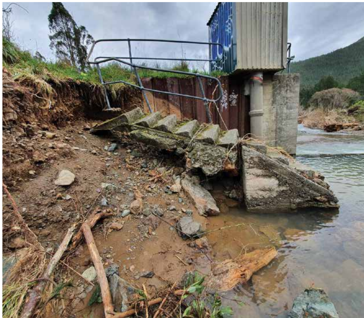
Picture 24: Collins at Drop Structure After the August 2022 Flood. Photo credit NCC
