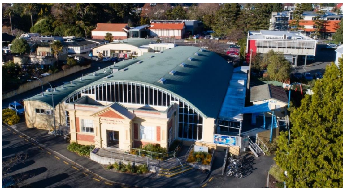
Figure 18: Riverside Pool, photo credit: RSL Consultancy Limited
