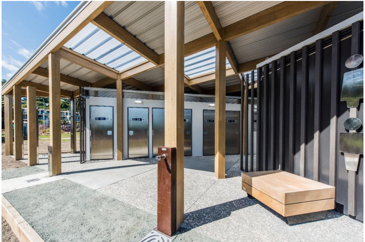
Figure 25: Toilets and changing rooms at Tāhunanui Beach
