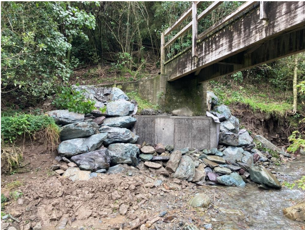
Figure 12: Barnicoat Track Bridge Abutment Repair, June 2023
