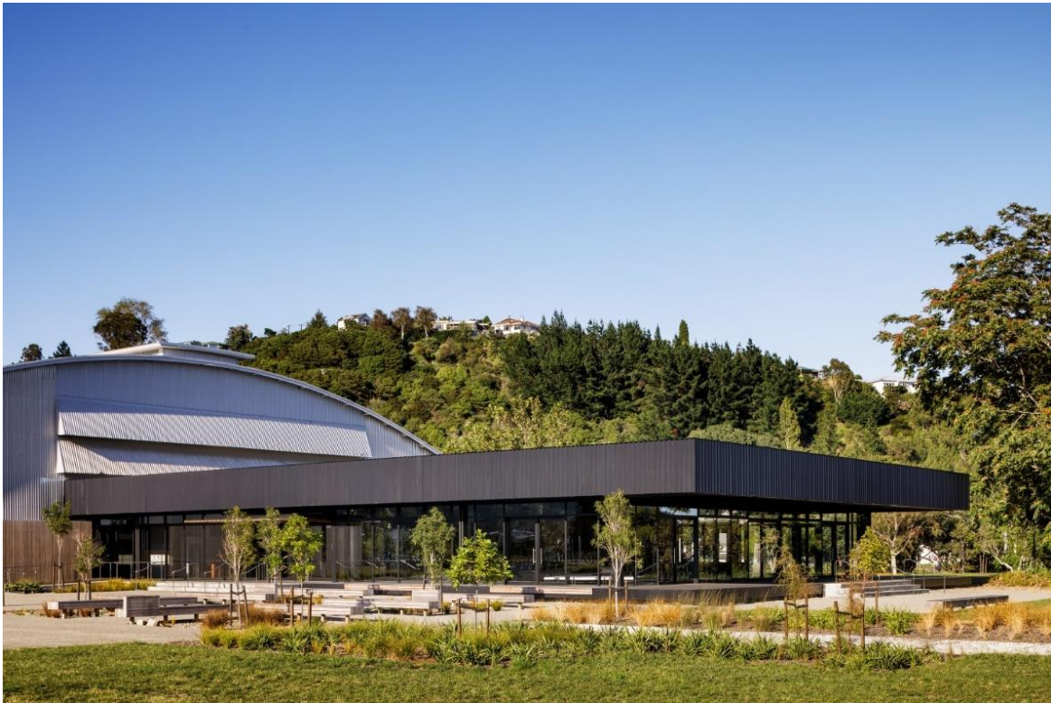
Figure 14: Trafalgar Centre northern extension
